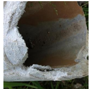
Example Asbestos Cement Pipe
