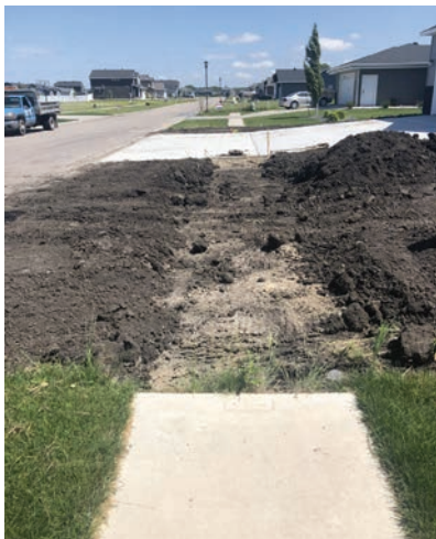
Photo 1: Lot 23 BLK 5 Brooks Harbor 2nd Looking South
