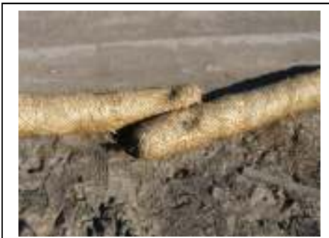
Overlapped wattle connection
