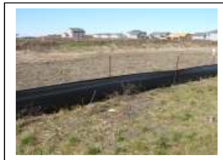
Standard silt fence
