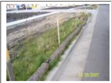
Straw wattles protecting curbline
