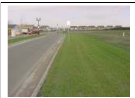
Filter strip protecting the curbline
