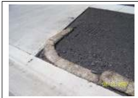
J-hooked upslope to contain sediment
