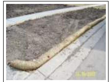
Residential site using straw wattles
