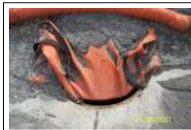
Gap allowing sediment to enter
