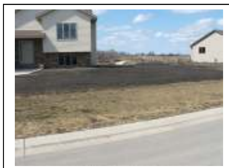
Filter strip used as a residential control
